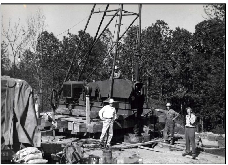
It early 1946 engineering contractors are conducting early surveys to determine the best site for Buford Dam. Core samples of granite were taken up and down the Chattahoochee River valley adjacent to the present site of Buford Dam. They had to be sure the site chosen for the dam would be able to support such a huge structure. Courtesy U.S. Army Corps of Engineers, Mobile District.
